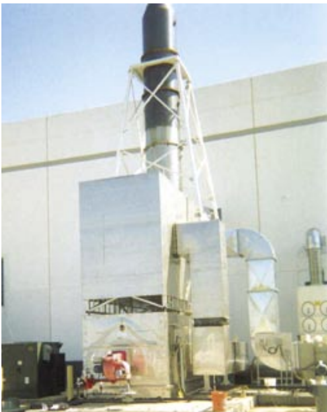
VOC - Recuperative Thermal Oxidiser 55, 000m 3 /hr - Dallas Texas
